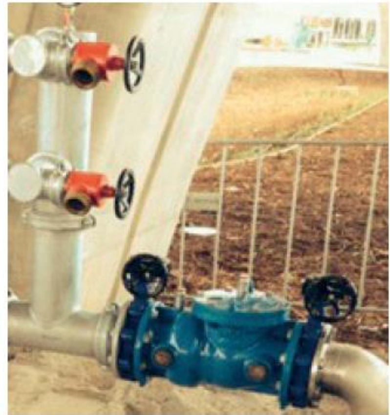
Image 4: Stainless steel upstream of SCVT
