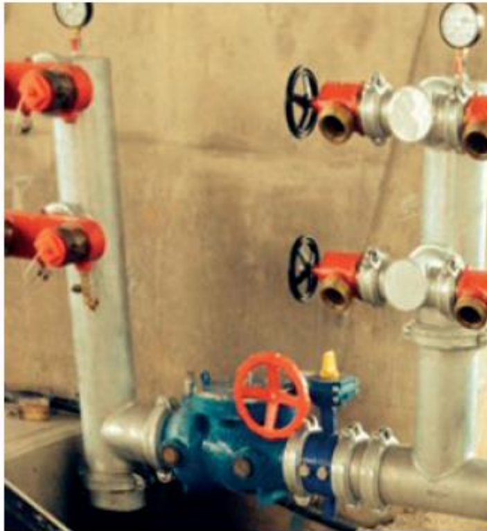
Image 2: Full-flow valve installed in 'H' pattern
