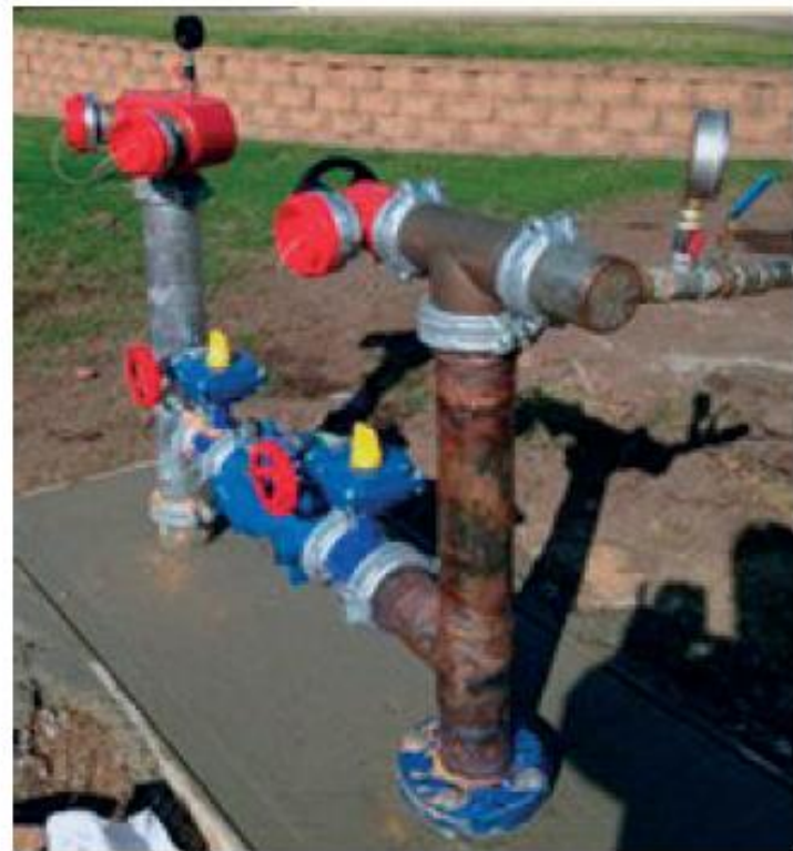
Image 3: Copper tube upstream of SCVT in 'H' pattern
