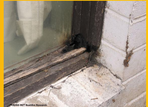
Poor timber condition
