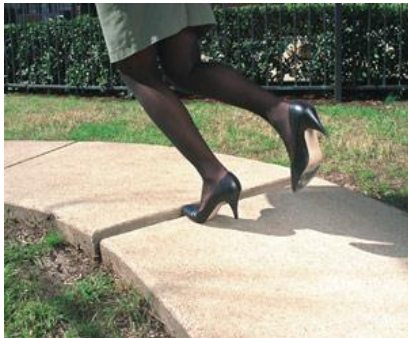
Problem: Sunken concrete path
