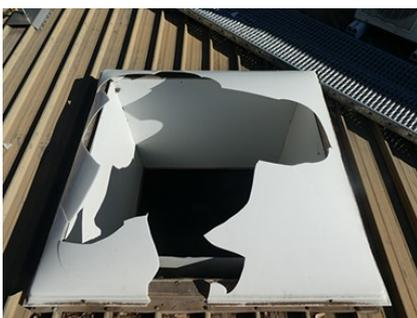
The first incident occurred when a contractor fell backwards through an unprotected skylight, falling 4.6m and sustaining multiple fractures. The contractor was inspecting anchor points on the roof at the time.
